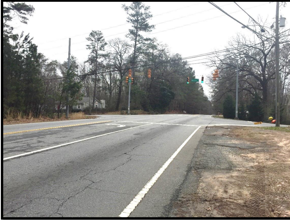
Photograph 3 – Northbound Lost Mountain Road at Bullard Road
