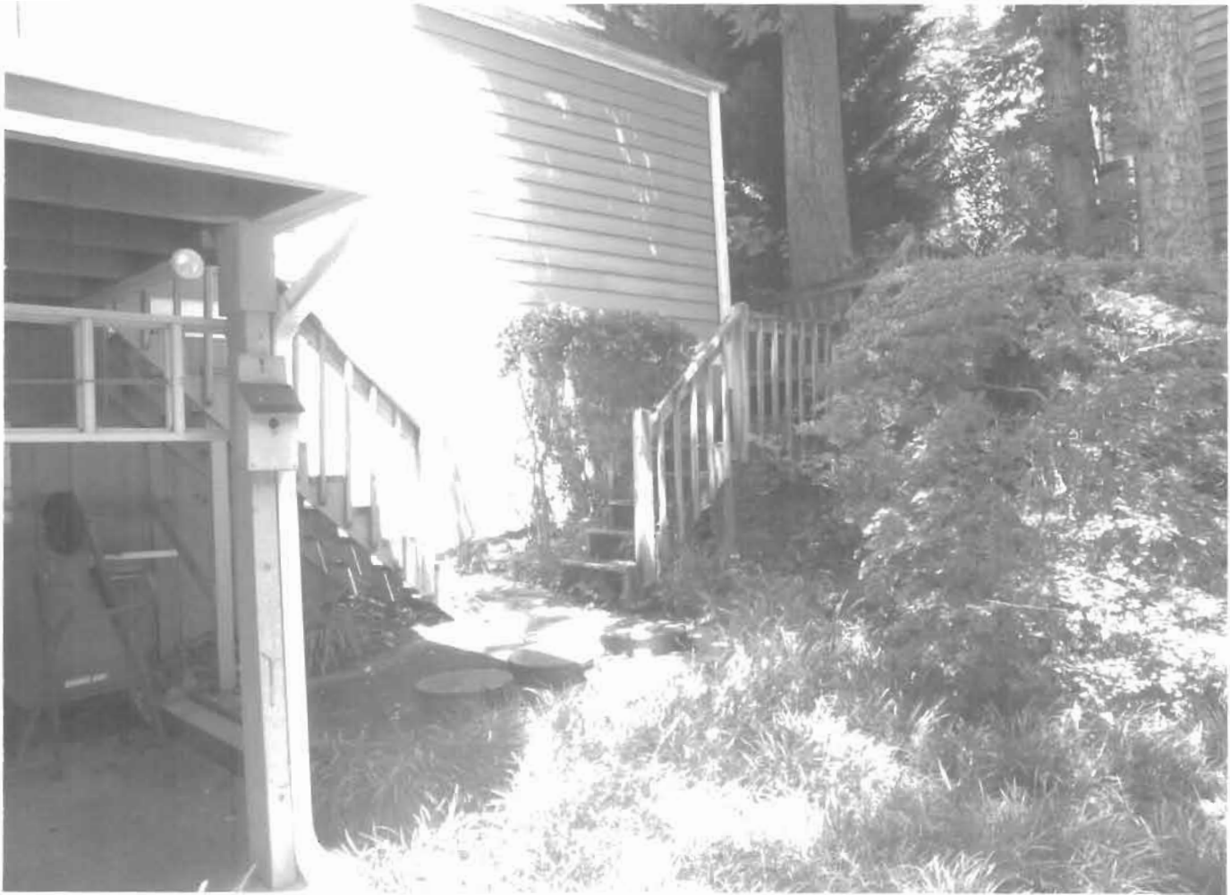
EXISTING LANDING + STAIRS
